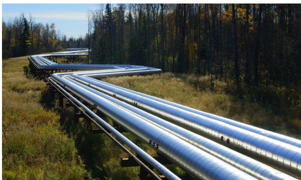
Tucker Thermal Project
