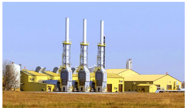
Edam East Lloyd thermal project
