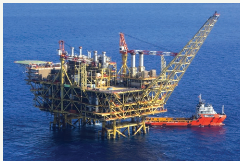
The Liwan Gas Project marked five years of safe and steady high-netback production in 2019.
